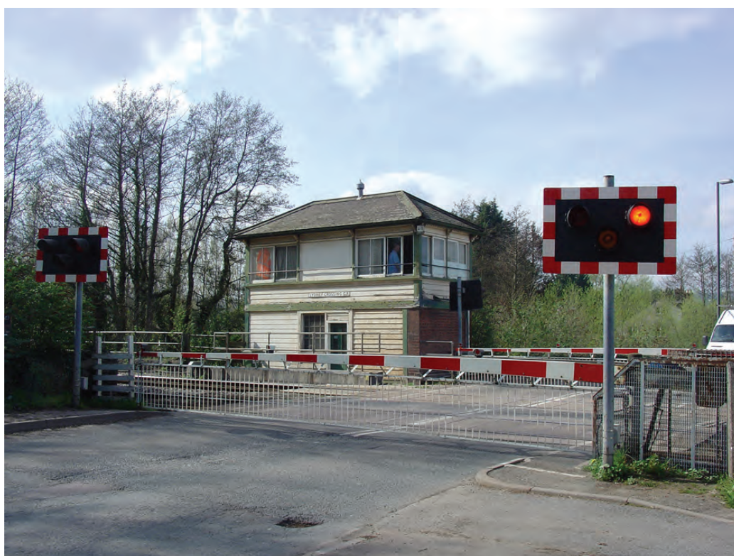
Lydney Road level crossing, Lydney, Gloucestershire, on the main line between Gloucester and Newport. A full-barrier level crossing controlled by a crossing keeper at the signal box shown in the picture. Credit: Rail Accident Investigation Branch.
