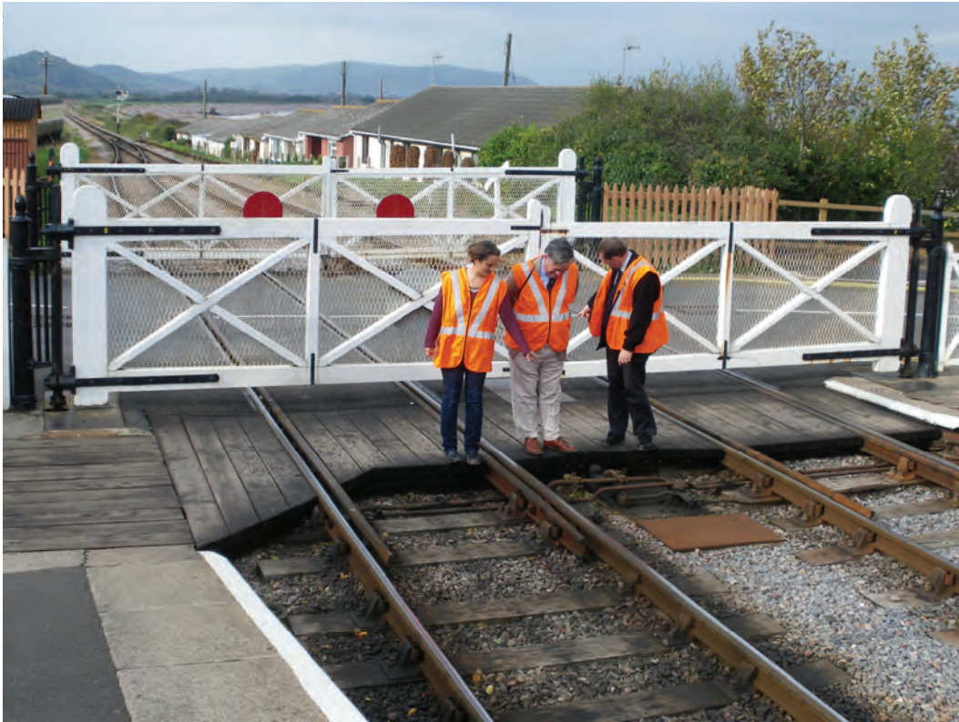
A traditional level crossing on a heritage railway. Members of the Law Commission team and John Jenkins, WSR Signalling Consultant, inspect the newly re-laid level crossing at Blue Anchor, one of the last crossings of this type in the South West. Credit: Ashleigh Keall.
