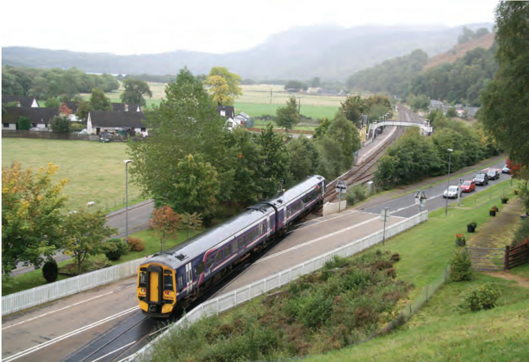
The automatic open (ungated) locally monitored level crossing (AOCL) at Garve Station on the Inverness to Kyle of Lochalsh line seen from the hillside. Credit: John Furnevel.
