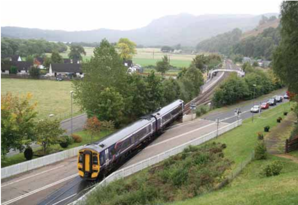
The automatic open (ungated) locally monitored level crossing (AOCL) at Garve station on the Inverness to Kyle of Lochalsh line seen from the hillside.
